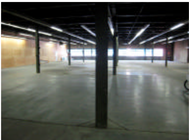
Ground Floor Space
